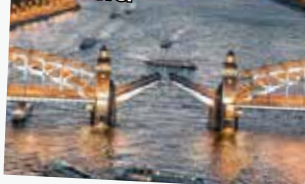
涅瓦河開橋 Open Bridge on Neva River
